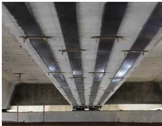
Application of ReArm Laminate to RCC Beam
